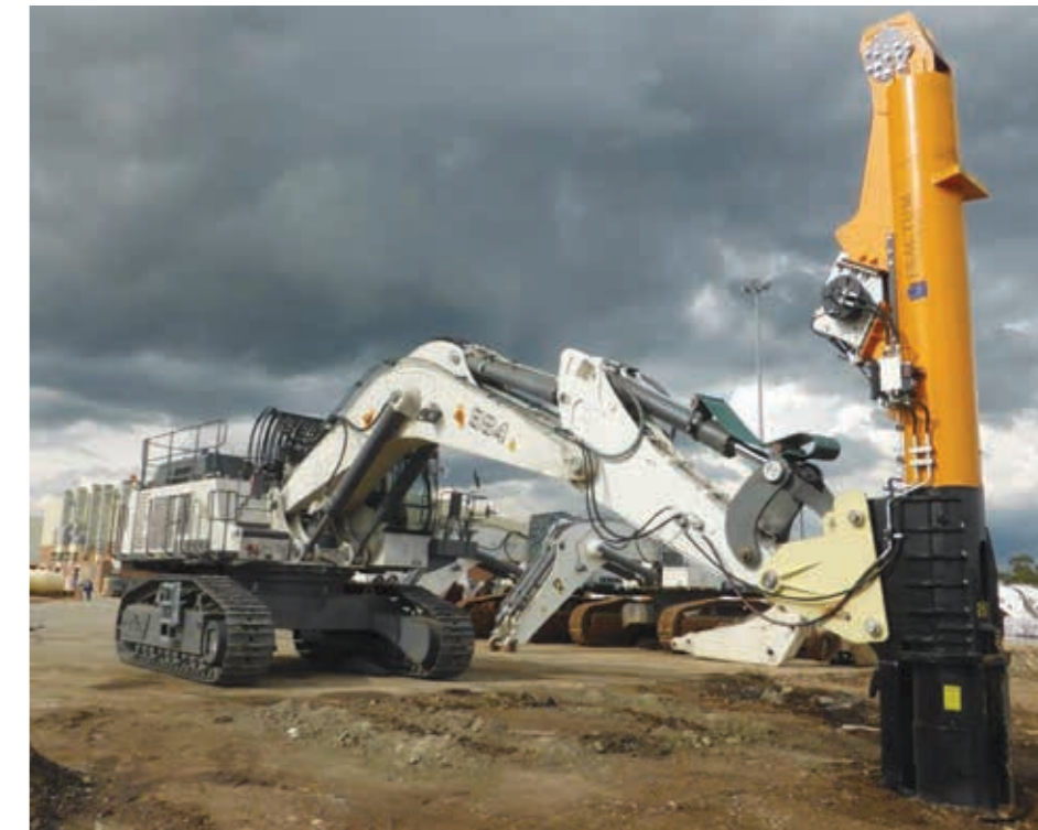
A Fractum 200 fitted to a Liebherr 984 excavator working at an iron ore mine.
